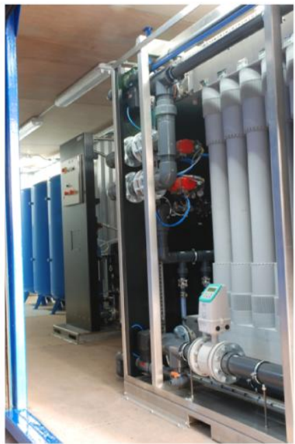
Internal Views of Tertiary Treatment Plant with Ultra-Filtration
