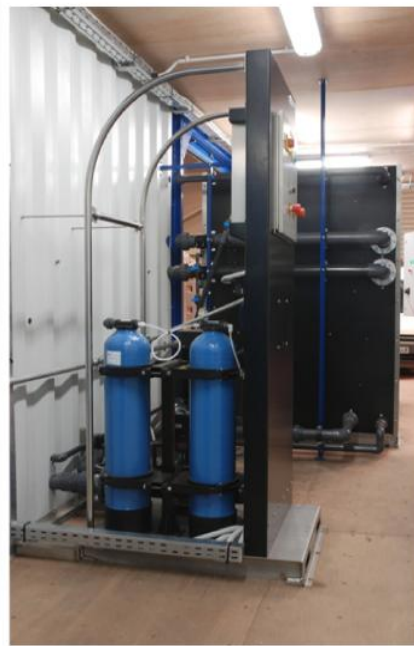
Internal Views of Tertiary Treatment Plant with Ultra-Filtration
