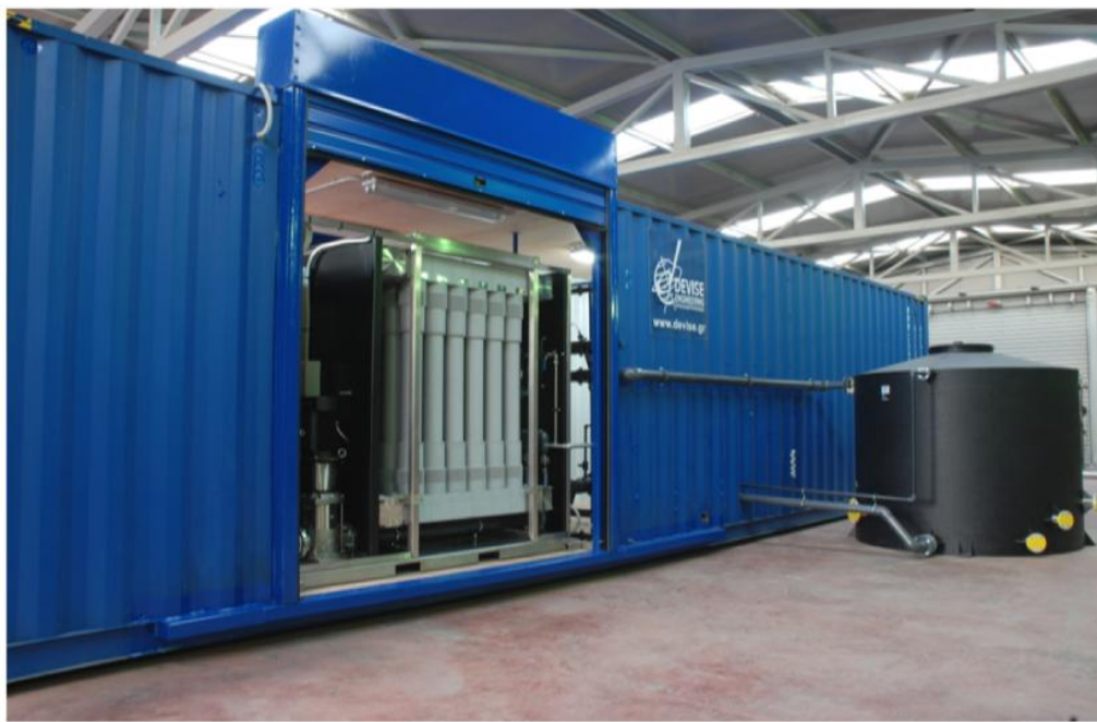
View of a Containerized Plant with Ultra-Filtration Membranes Capacity: 900 m 3 /day for tertiary Treatment of Wastewater Capacity: Up to 1800 m 3 /day for Potable Water Treatment
