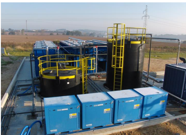
Multiple Packaged Bio Plants operating in Parallel in the Wastewater Treatment Plant of the "Colgate-Palmolive" Factory
